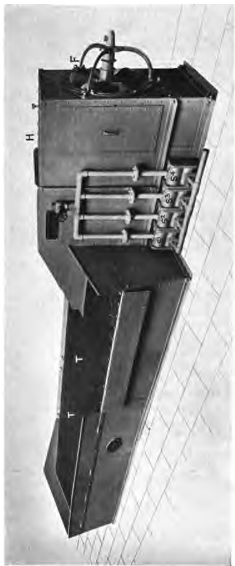
Fig. 15 HATTERSLEY-PICKARD TABLE DRYING MACHINE
